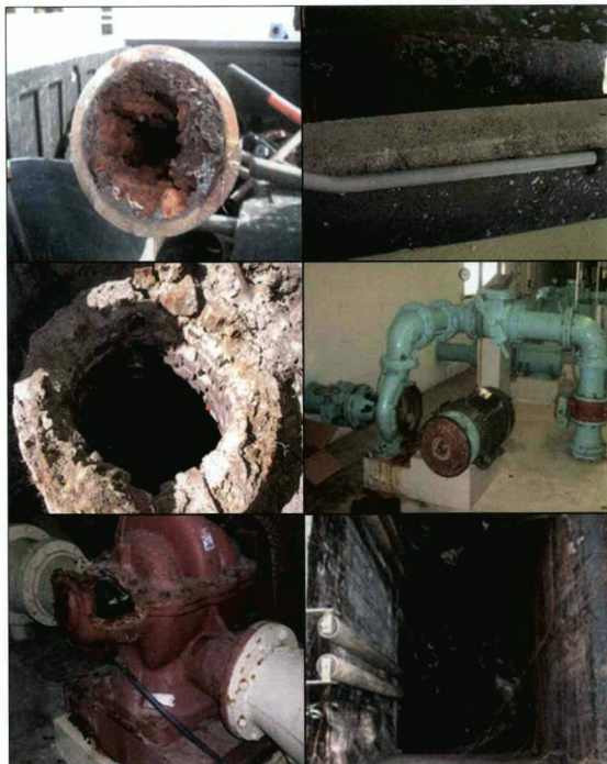
Using photographs of a utility's renewal and replacement needs can graphically illustrate to regulators and the public the reasons for raising rates. Top left, a severely tuberculated water main; top right, a hydrogen sulfide-damaged pipe; center left, a deteriorating manhole; center right, aging water plant infrastructure; bottom left, a corroded well pump; bottom right, aging lift station infrastructure.
